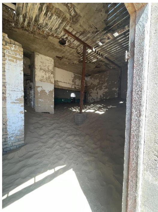
A typical sand-filled interior in Kolmanskop.
